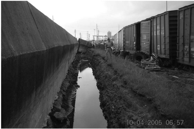
Fig. 2. View of the I-wall failure at the Port of New Orleans, from the inboard side, showing the trench scoured behind the I-wall by overtopping flows
