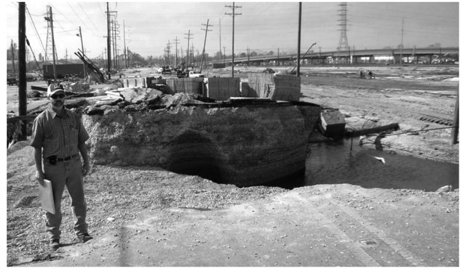
Fig. 3. Southernmost breach along the west bank of the IHNC, showing the lightweight shell-sand fill of the remaining intact levee embankment section adjacent to the eroded breach
