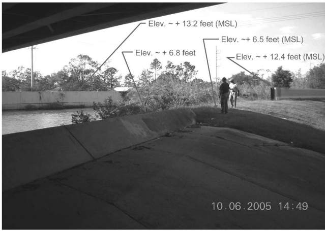
Fig. 4. Side view of the “gap” in the flood defenses at the south end of the Orleans canal
