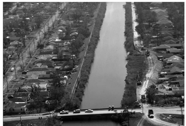
Fig. 7. Oblique aerial view of the breached (North Breach) section on the west bank of the London Avenue Canal (on the right side of the photo, which is taken looking to the south), and the distressed section on the east bank (on the left in this photo)
